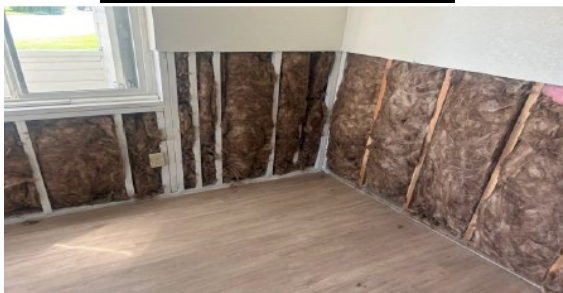
(3) New insulation installed
