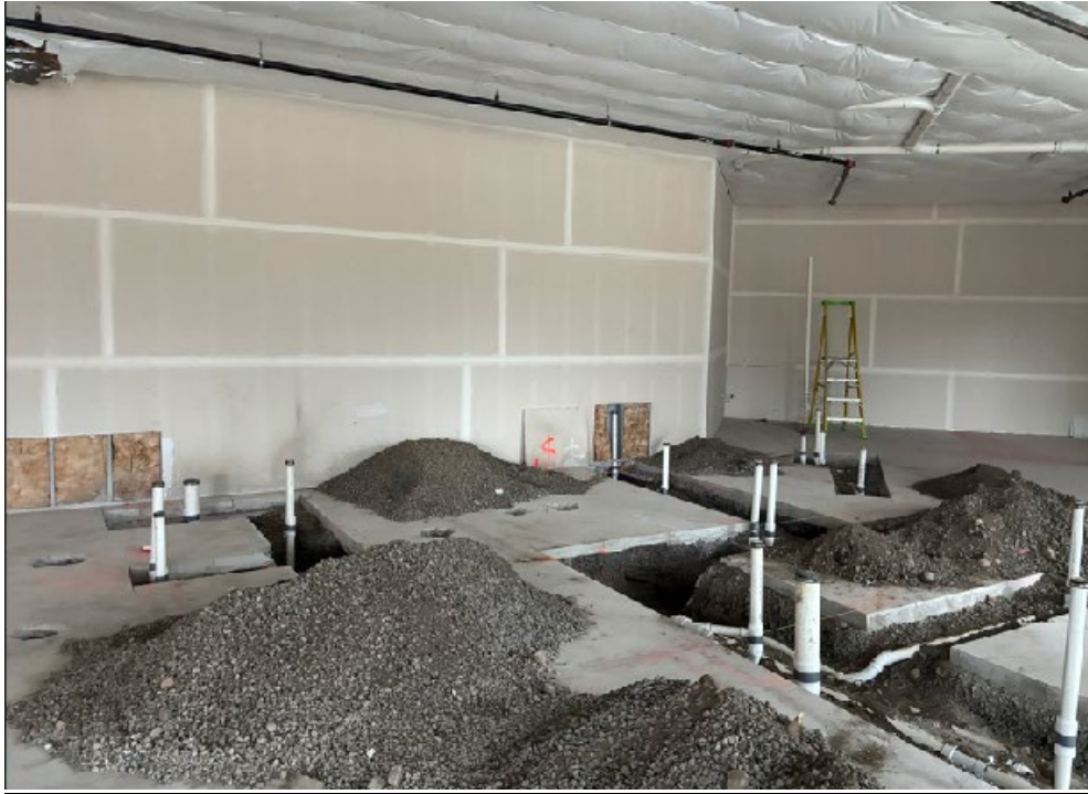
Photo: New Below Slab Plumbing
