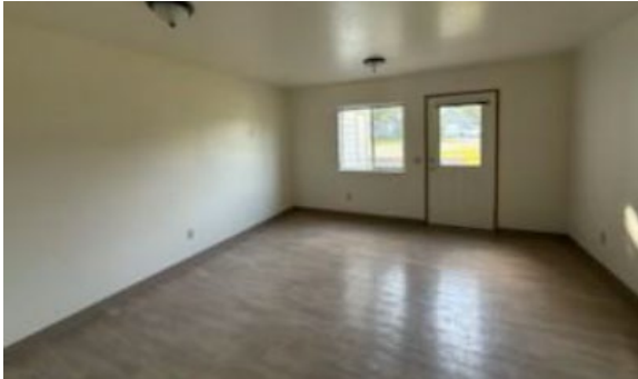
(1) Before work began
