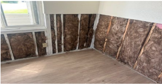
(3) New insulation installed
