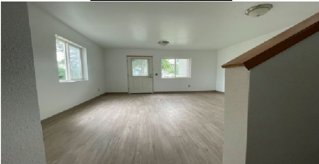
(5) Final paint and flooring complete
